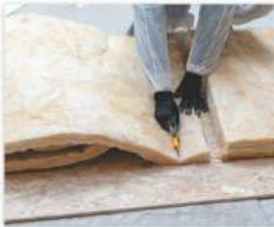
Rockwool Stuffing (Thermal Installation)
